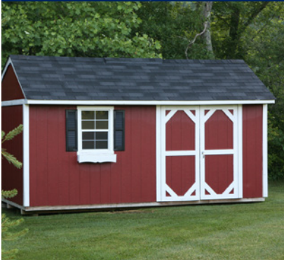
Undercoat Before Paint
