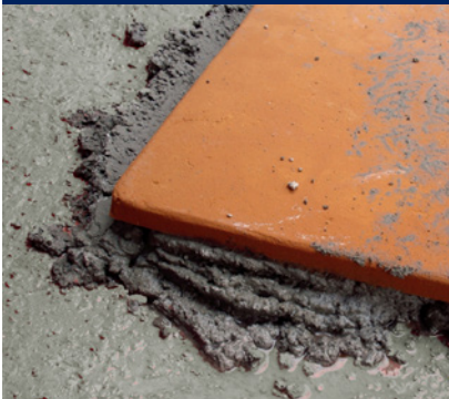
Undercoat Before Tile Mortar
