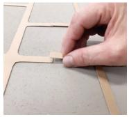
Overlap the tips of adjoining stencils slightly during placement for a continual clean pattern and less leakage.
