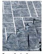
Remove the stencil as soon as the coating is dry and will support your weight. Peel it up with care to avoid breakage. With the dry coating on the stencil surface, it will become even more durable and water-repellent, allowing it to be re-used.
