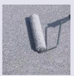
3) Pour out a 10-12" puddle. Start at one corner of the installation surface and work your way out from there. Pour out more puddles as required.
