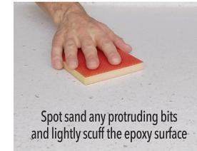
Spot sand any protruding bits and lightly scuff the epoxy surface
